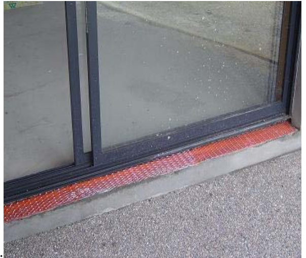
☞ renderlok secured to masonry with approved concrete nails. - (15mm length preferred)
