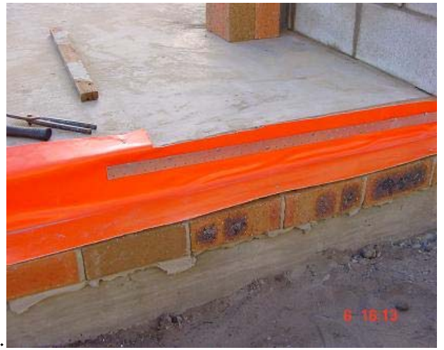
☞ if tiling is to extend to slab edge Kordon TB is installed as shown - secured with gal hoop-iron/strapping.
